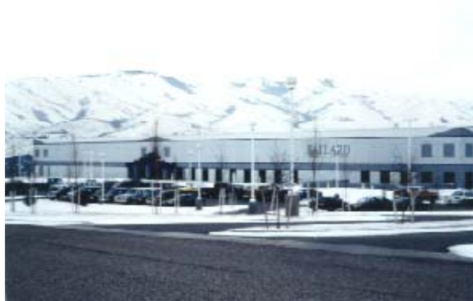
Ballard Medical – Light industrial development.
