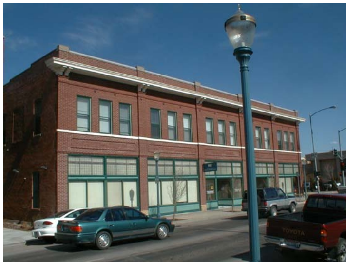
The Eagles Building on Arthur Street was recently renovated. Office space is provided on the ground floor and affordable rental housing is provided on the upper floor.
