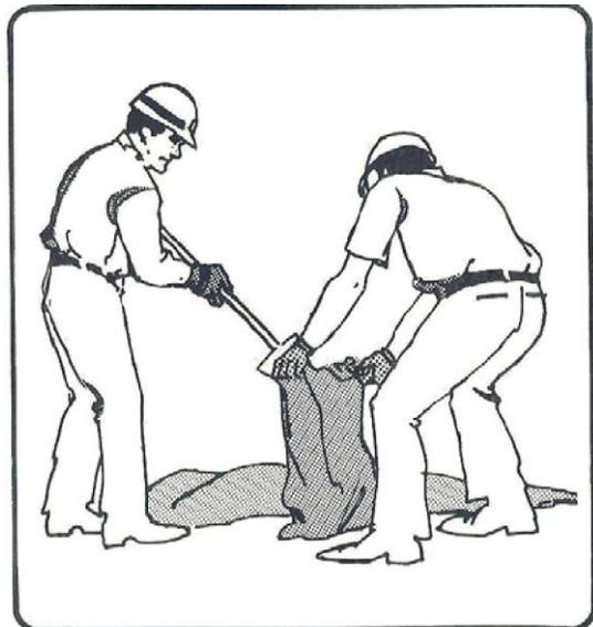
For large-scale operations, filling sandbags can be expedited by using bag-holding racks, metals or plastic funnels and power loading equipment. However, the special equipment required is not always available during an emergency.
